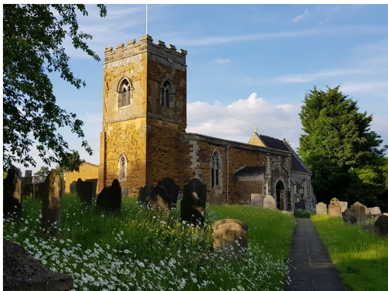
Figure 4: St Luke's Church
